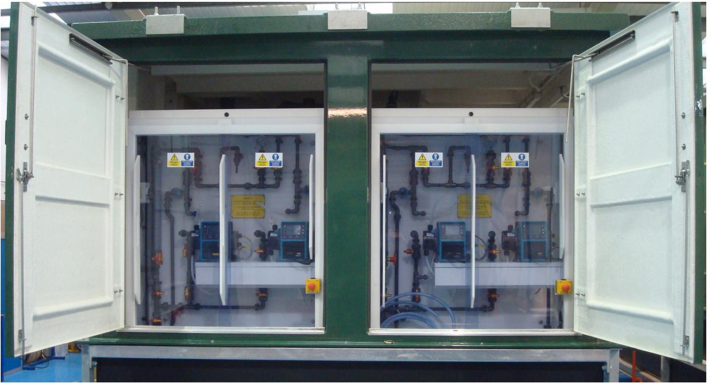
That project took an important step forward this year, with the installation of the first of a new range of modular chemical dosing systems at the company's wastewater treatment site at Chilcompton in Somerset. The system was designed, manufactured and installed by chemical dosing specialist WES, which worked in close collaboration with Wessex Water and its engineering partners to develop and refine the unit.
